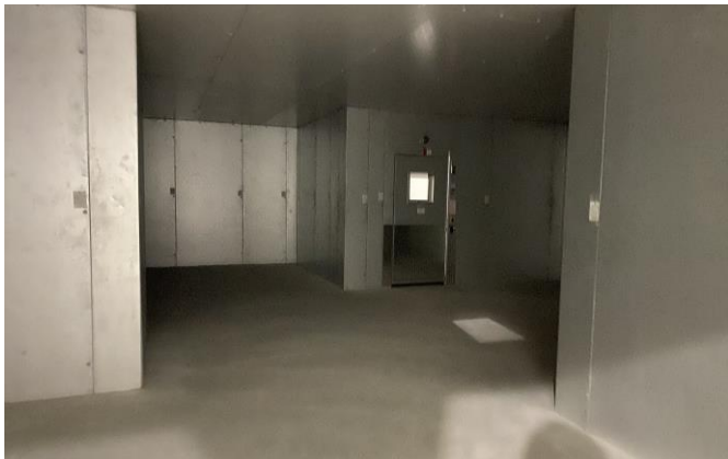
Kitchen cooler and freezer is assembled 02/15/2023
