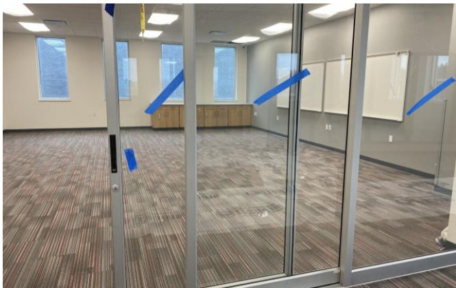
Sliding glass doors in classrooms are installed 02/15/2023
