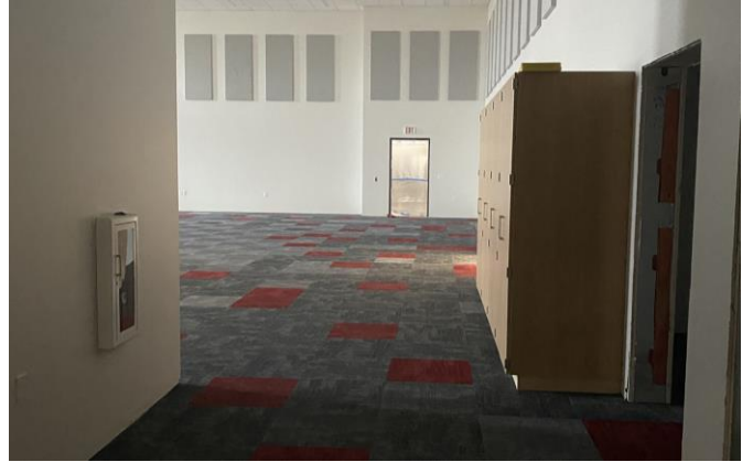
Carpet installed in music rooms 02/15/2023
