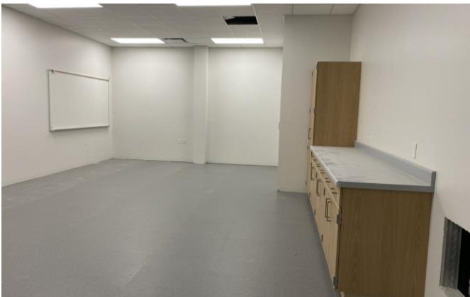
Completed casework and rubber flooring 02/28/2023
