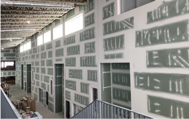
Spirit concourse ready for paint 02/17/2023
