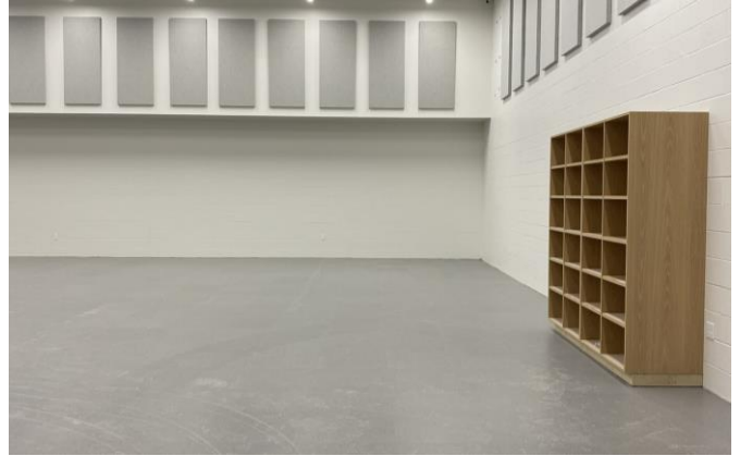
Rubber flooring installed in choir room 02/28/2023
