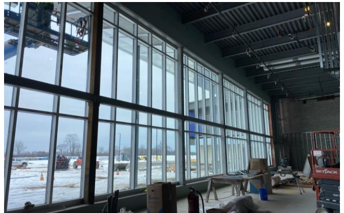
Auditorium lobby window glass is installed 02/28/2023
