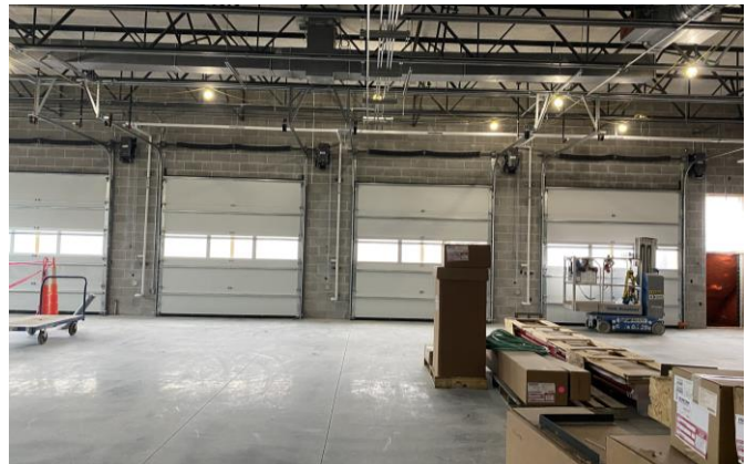
Overhead doors in auto shop installed 02/15/2023
